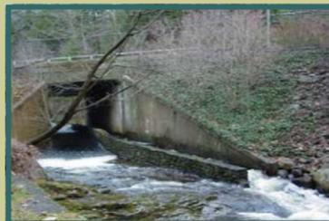
**Fishways** can be utilized where baffles or gradient control weirs are not viable retrofit options.
