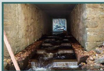
**Baffles** can be used to facilitate fish passage by creating a series of pools with drops to increase water depth and decrease water velocities. Baffles can increase debris clogging and accumulation and therefore require periodic maintenance.
